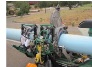
•A closer look at the PVC heat fusion device. (IEC)
