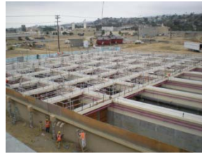
•IBWC waste water treatment plant construction site. (Malcolm Pirnie)
