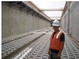
•Takesi (left) from Malcolm Pirnie is inspecting the Fine Bubbles Diffusers in AST Basin #2 at IBWC. Takesi (right) is at his desk electronically linking RFI documents to contract documents
