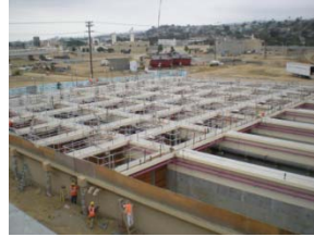
•IBWC waste water treatment plant construction site. (Malcolm Pirnie)
